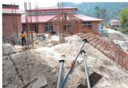
CSSD new building is being progressed
