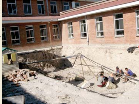
The 100,000 litre underground under construction at HRDC
